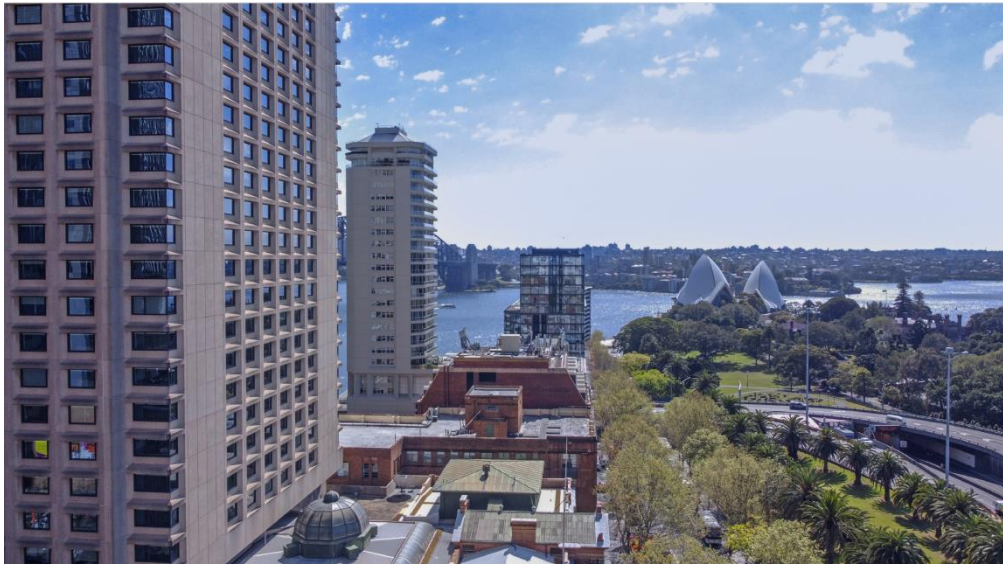
Figure 15: Drone photo from northern elevation of the Astor building facing north
