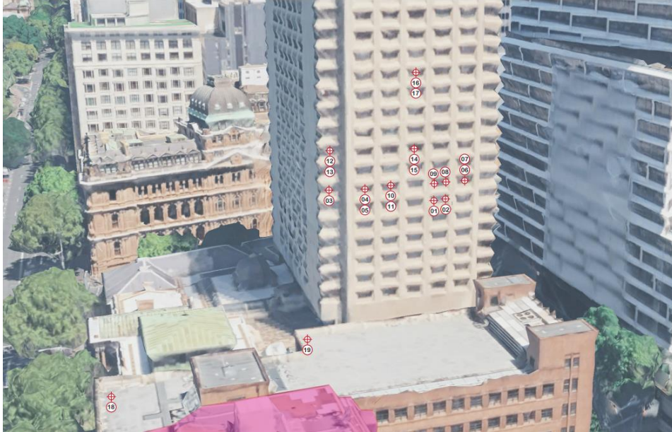
Figure 18: Northern elevation of the InterContinental Hotel showing rooms that were assessed as part of the supplementary Visual Impact Assessment
